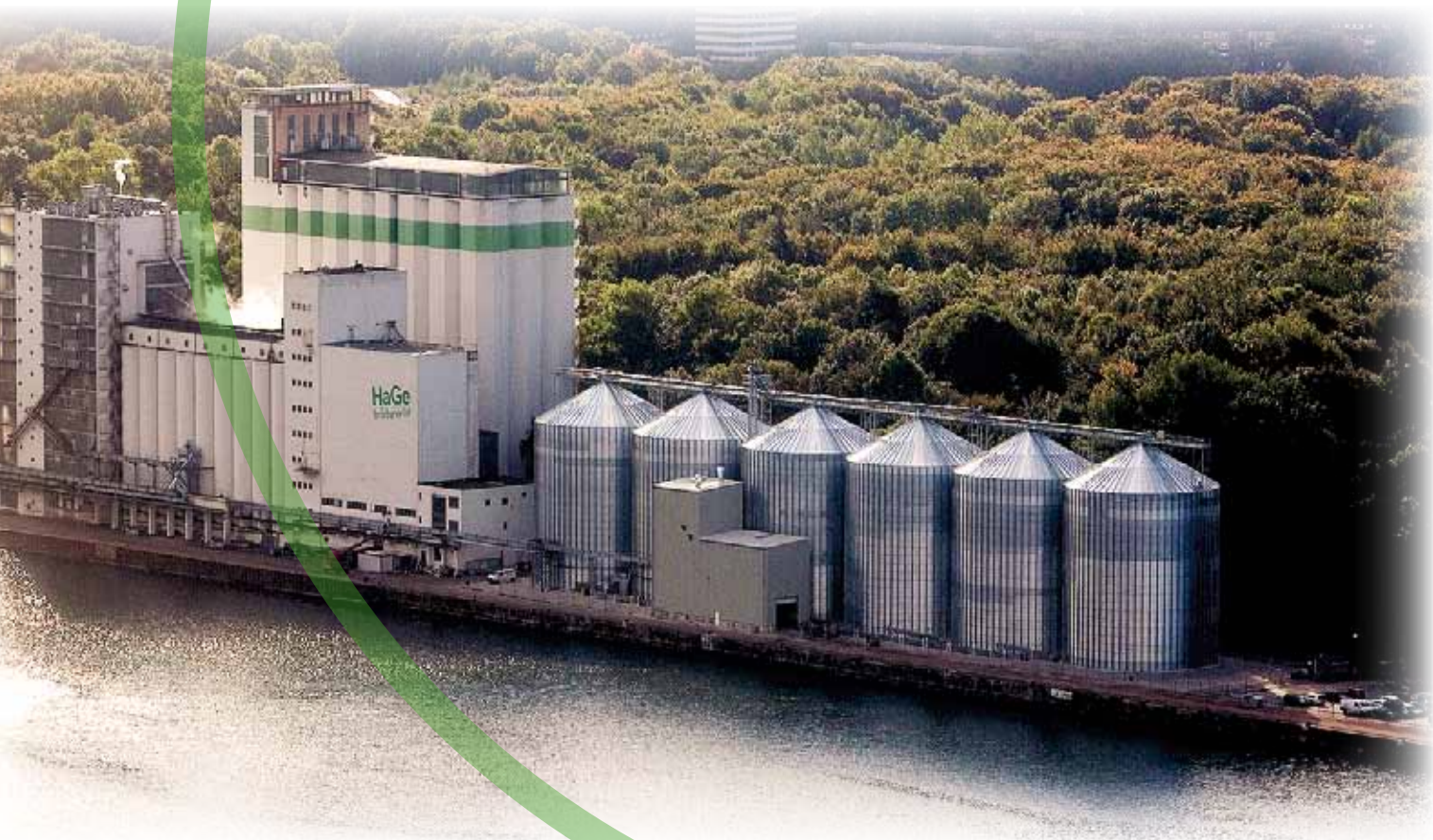
SKN Silo Kiel-Nordhafen, capacity for grain 110.000 tons
